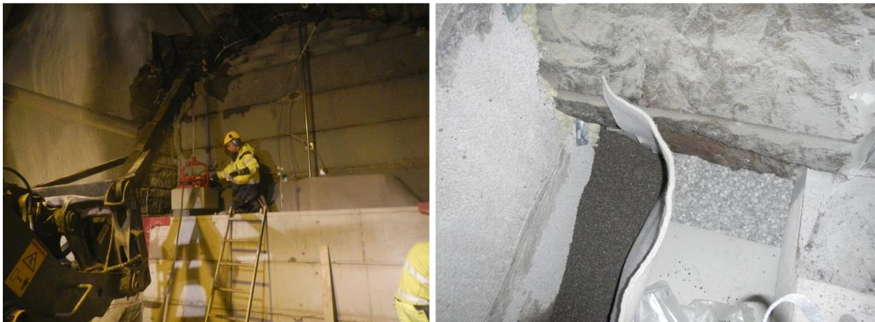
**Figure 2.** *LEFT: emplacement of bentonite block in the sealing. RIGHT: filter section (LECA-beam and macadam) together with geotextile, bentonite block and bentonite pellets.*
