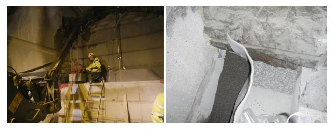
*Figure 2. LEFT: emplacement of bentonite block in the sealing. RIGHT: filter section (LECA-beam and macadam) together with geotextile, bentonite block and bentonite pellets.*
